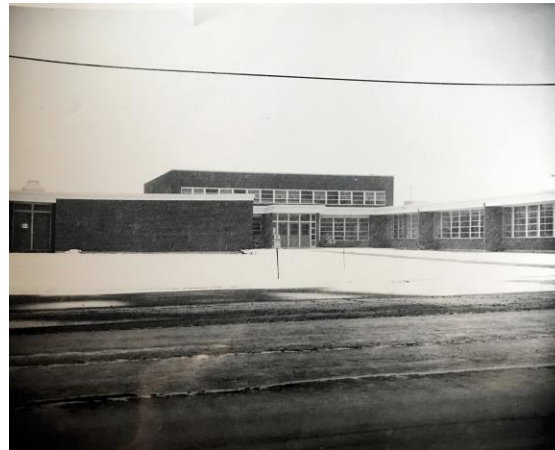
Barton Elementary School
