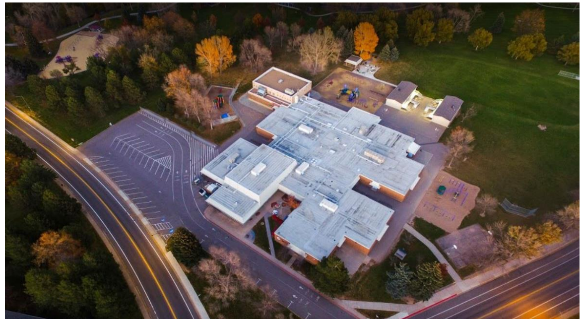
Aerial photo of Riffenburgh Elementary (right)
