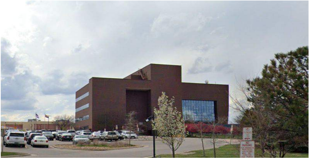
Arapahoe County Jail (additions and alterations): 7375 S. Potomac St. Centennial, CO
