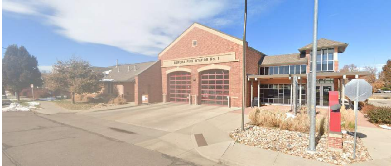
Aurora Fire Station: 9801 E. 16th Ave. Aurora, CO
