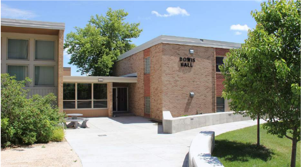
Northeastern Junior College, Women's Dormitory - Dowis Hall: 100 College Lane, Sterling, CO
