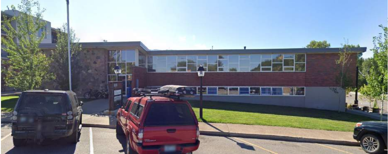
Yampa Valley Electric Association Building: 32 10th Street Steamboat Springs, CO
