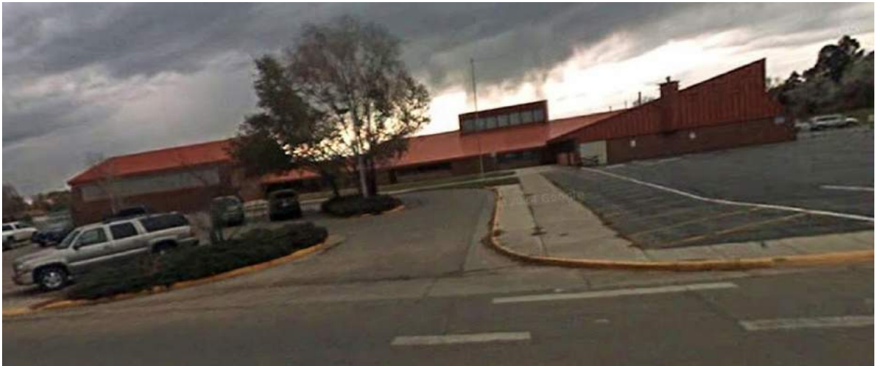
Sunset Elementary School: 800 W. 7th Street Craig, CO
