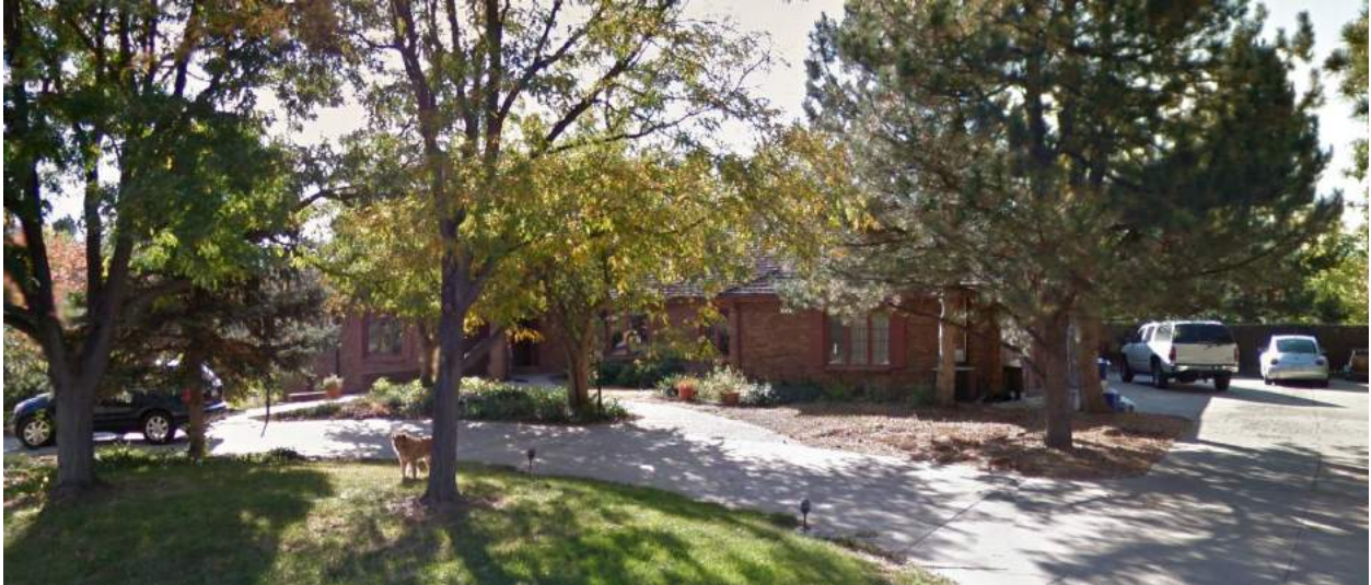
Miller (Mr. Mrs. Martin P.) residence: 580 Front Range Road Arapahoe County, CO
