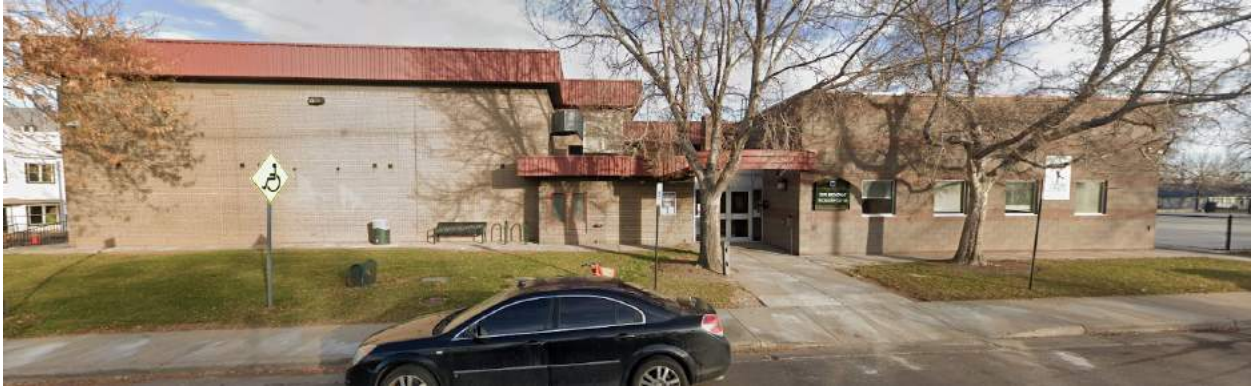
Stapleton Community Center: 51st Ave. and Broadway Denver, CO
