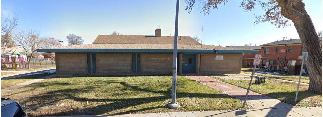
Quigg-Newton Community Center: 4430 Navajo St. Denver, CO
