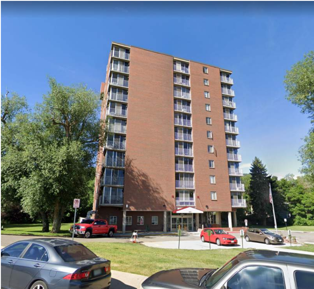
Apartment Building: Arapahoe Ave. at Lincoln Place Boulder, CO
