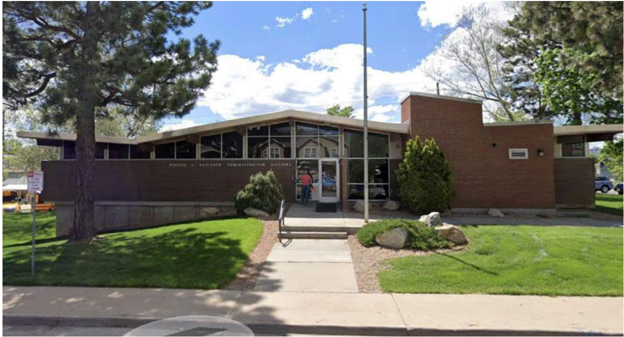
Englewood Public Schools Administration Building: 4101 S. Bannock St. Englewood, CO
