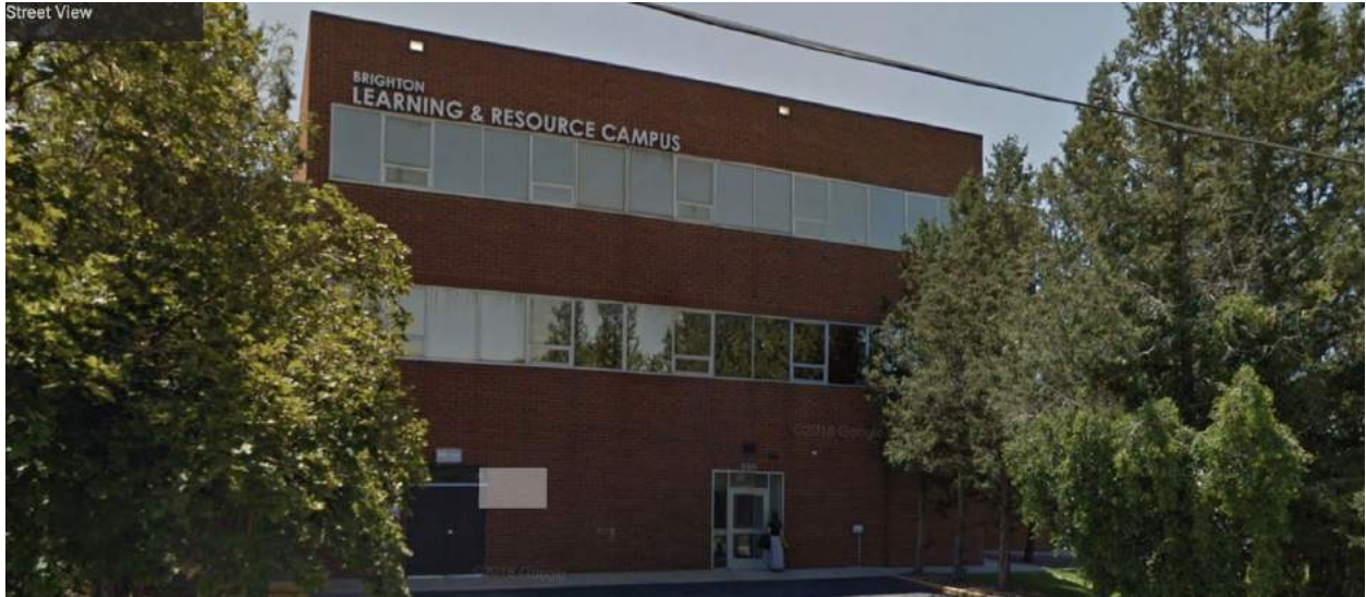
Brighton Community Hospital: 1850 Egbert St. Brighton, CO
