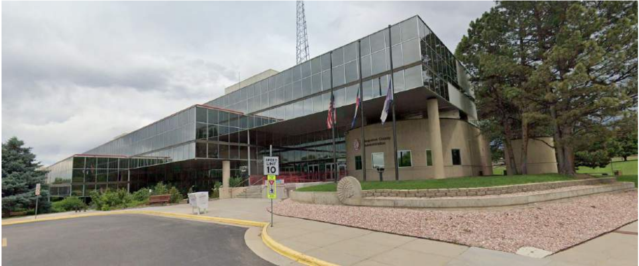
Arapahoe County School District Number 1, Administration Building: 5334 S. Prince Street, Littleton, CO
